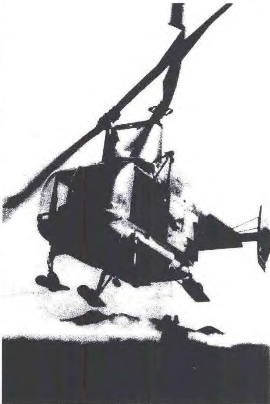
First arriving in Vietnam on October 20, 1964, the Kaman HH-43 Huskie was the first helicopter designed specifically for rescue, but its 140-mile range was inadequate.
