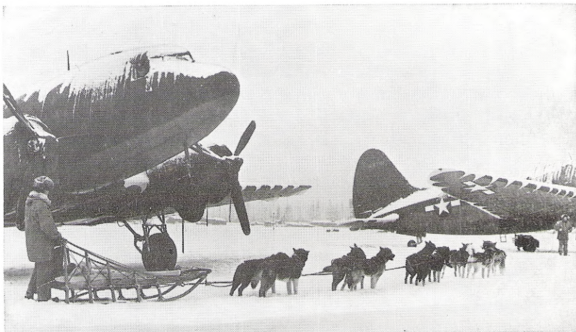
MAINSTAYS of units in the far north were the ubiquitous C-47 and superb dog teams trained to reach otherwise inaccessible crash sites.
