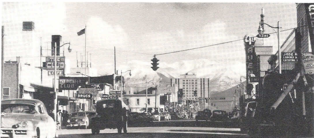
4th Ave., Anchorage, Chugach Mountains in background.
