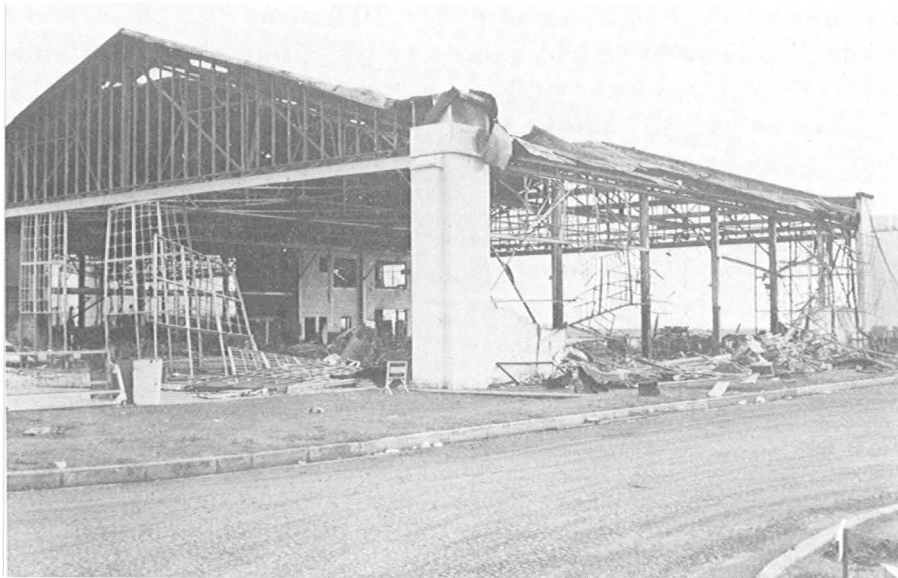
Above, when the flames died down and the smoke cleared, all that remained was the skeleton of Hangar 3; and below, total devastation in Hangar 3. (Joe K. Harding)
