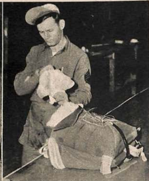
S/Sgt. Amos A. Owen packing a parachute on a table that service men had made out of latrine screen, which they attached to iron fence posts and welded, brushed and polished.
